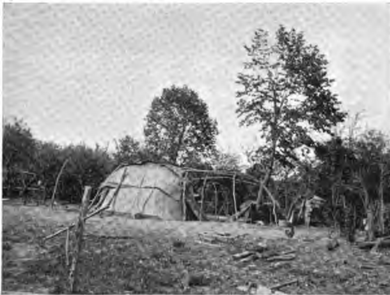
Showing the frame-work of a wickiup.
